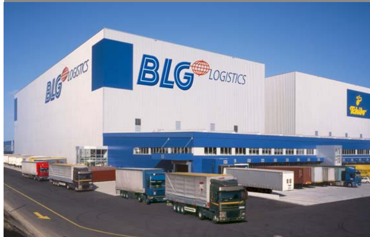
Hochregallager der BLG Logistics Group
